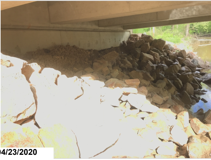
Bent 4 riprap starting to slide into channel, riprap was placed in 2019 from flooding.
