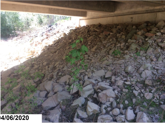
Slope protection at bent 2 end
