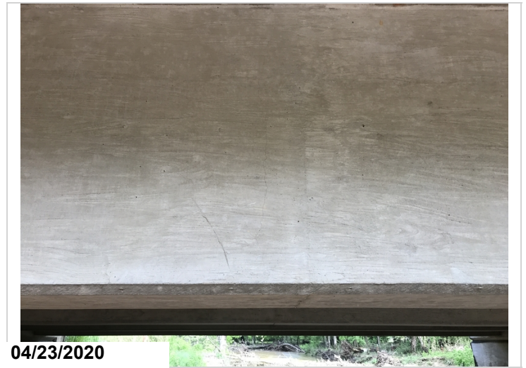
Hairline cracks
