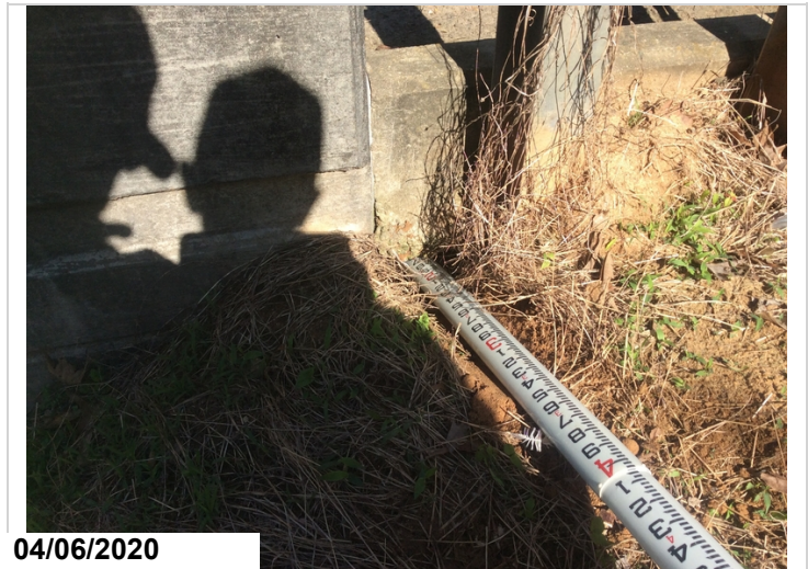
2 ft erosion left side behind back wall beginning of bridge
