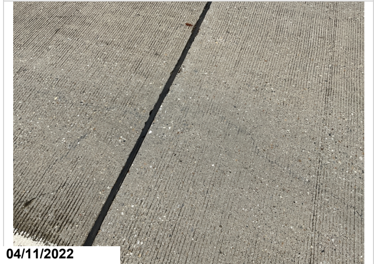
04/22 cracking in top of deck
