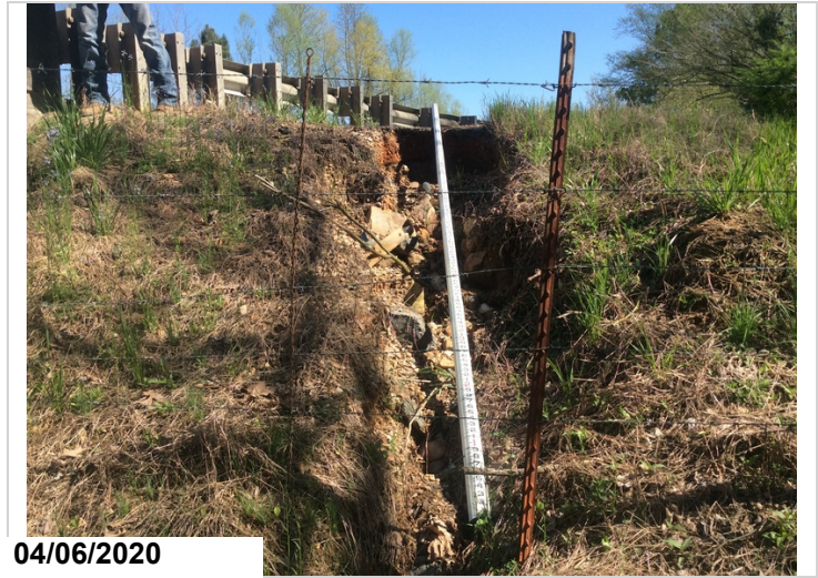
EROSION BEGINNING OF BRIDGE LEFT SIDE. 13 ft.
