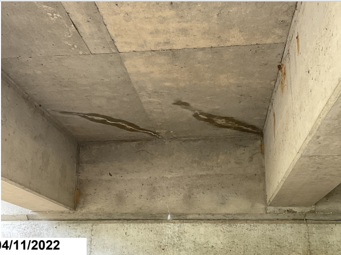
04/22 efflorescence photo
