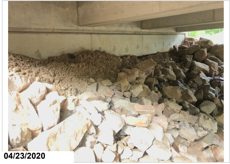
Bent 4 riprap starting to slide into channel, riprap was placed in 2019 from flooding.
